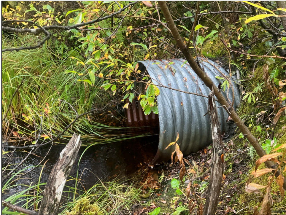
Figure 3.—Culvert upstream of the road at waypoint 1242.
